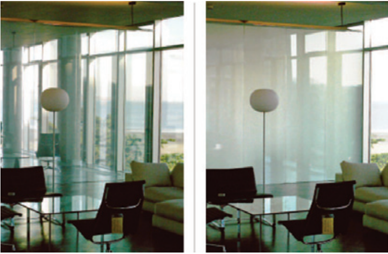
FIG 1.5: Now you see it, now you don't: smart glass can be configured to become opaque automatically ( http://bkaprt.com/rwd/7/ ).
